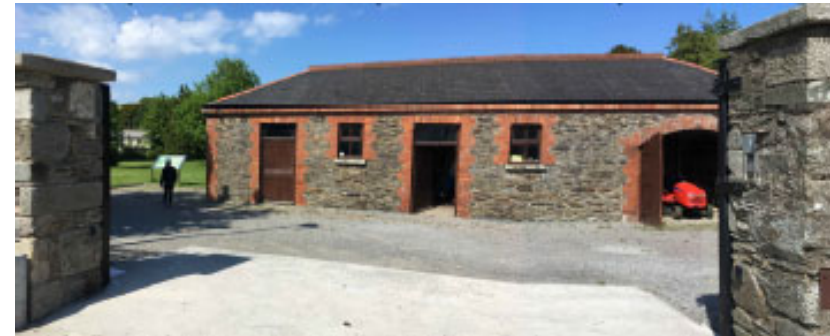
Looking at the Coach House from Abbey Street, depicting view impediment
